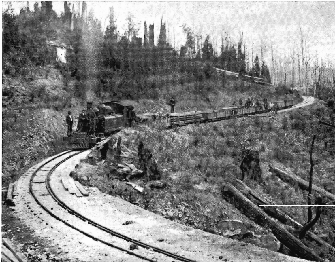
View from 27 miles 16 chains, looking north, during the construction of the line. Like other ranges in southern Victoria, the Otways were rich in stands of magnificent mountain ash and other timbers. The remains of some of these giants can be seen in this picture.
