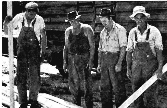
BEALIBA (9) gang won first prize in the Ballarat District for the best kept length with rails over 75 lb. Left to right: Repairers J. V. Milley, M. Milley, and A. J. Jenks, and Ganger A. T. Whitford (Repairer S. R. Holt was not available when this picture was taken).
