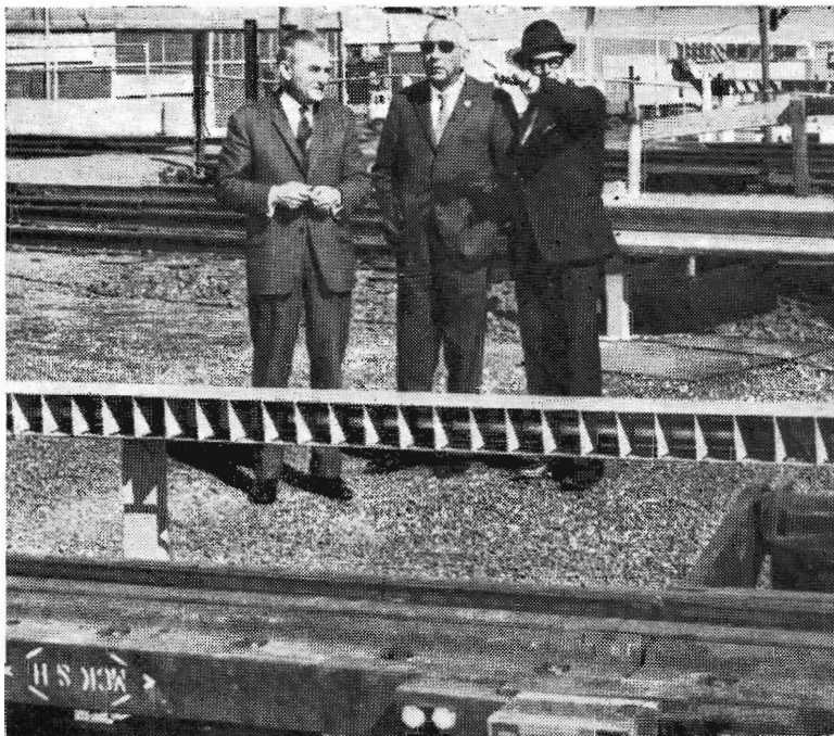
Automatic shunting, with computer controlled retarders, automatic switching, and radio signalling, started in Melbourne's freight terminal on Tuesday, August 25, when 10 of the 32 tracks in the rebuilt yard were brought to use. The following week, another six tracks came in, and the yard is expected to be officially opened towards the end of next month. Introduction of automation was watched by Commissioners, senior railway officials, the Chief Secretary and Deputy Premier (Sir Arthur Rylah), and representatives from the Press and TV. Here, Sir Arthur Rylah (centre) listens to details of retarder operation explained by Mr. Commissioner L. A. Reynolds (right). At left is Mr. E. P. Rogan, Deputy Chairman.
