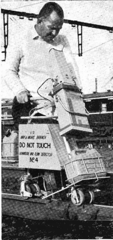
Important aids to rail safety are the Rail Flaw Detectors. One of the five ultra-sonic Miniature Rail Flaw Detectors in service is shown above.
